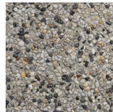
Exposed aggregate driveway, Beachside
